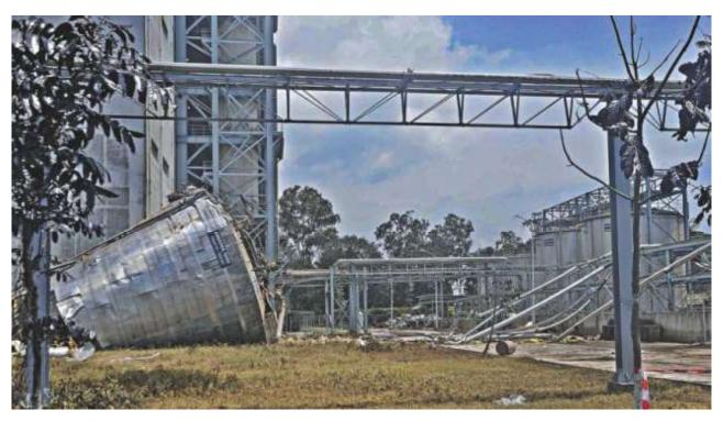
The damaged gas tank and pipes of DAP Fertiliser Company Limited in Anwara upazila of Chittagong. An explosion at the factory on Monday night caused the damage. Photo: Anurup Kanti Das
